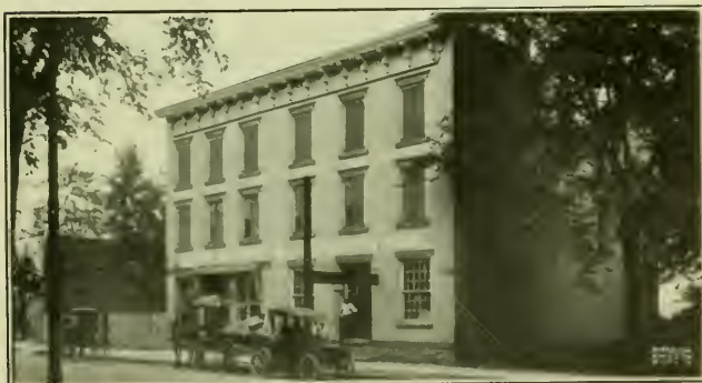
BROWN & DRESSEL, PLUMBING.
